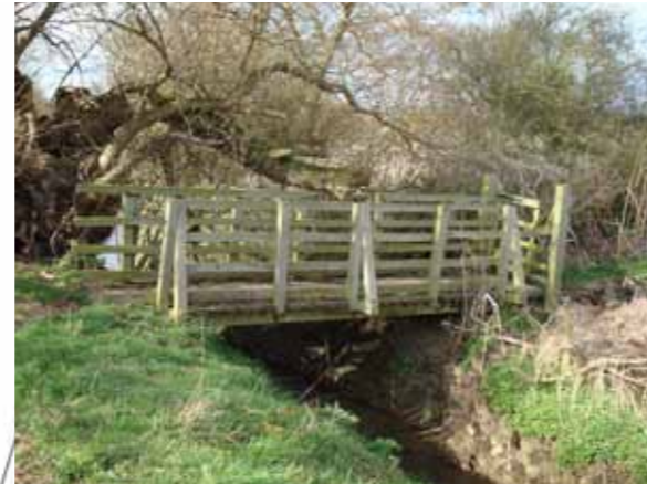
View of existing bridge
