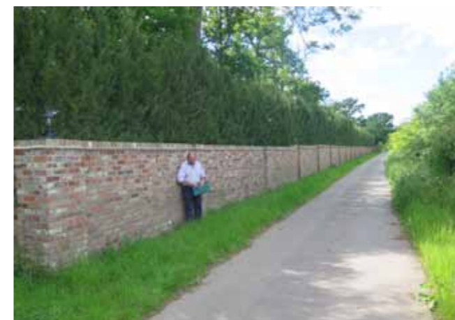
Existing Estate wall
