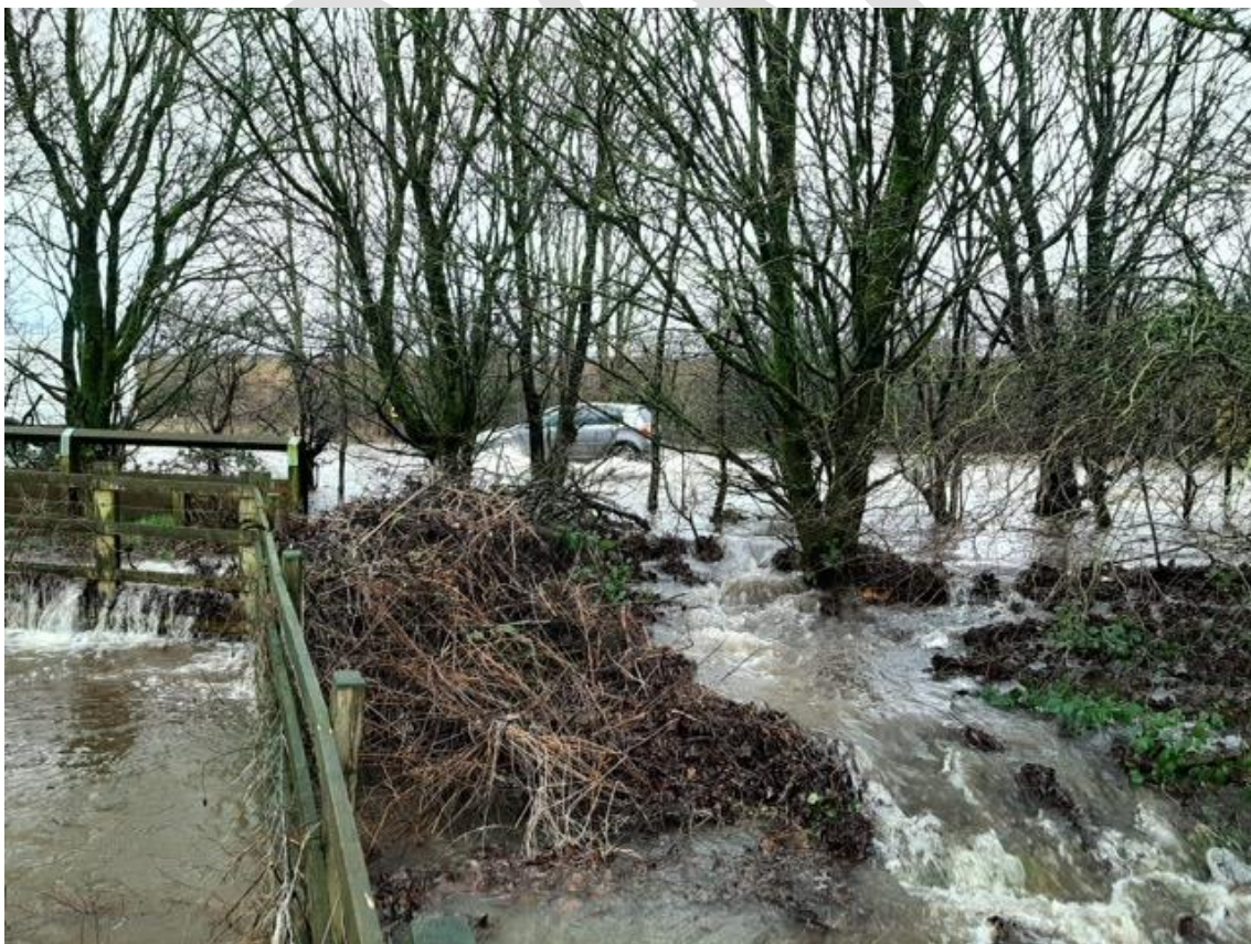
Figure 15: Gildersleets - floodwater by-passing bund
