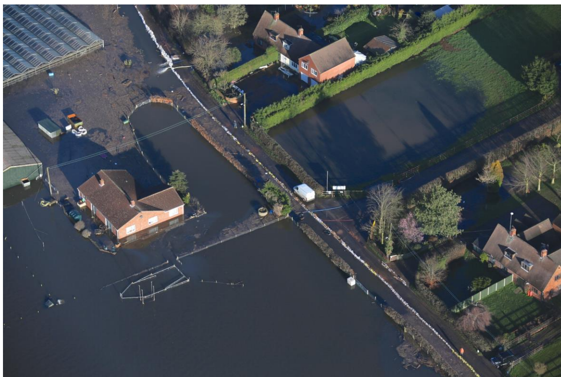
Figure 18: West Bank - Makeshift Defence
