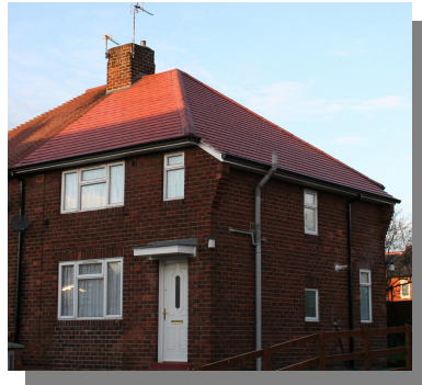
508 new roofs 441 new heating systems 59 new kitchens & bathrooms
