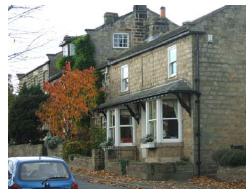
Roof height variation add interest to the Conservation Area.
