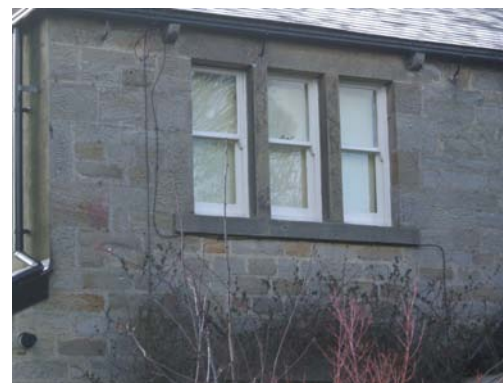
An example of stone mullioned windows.
