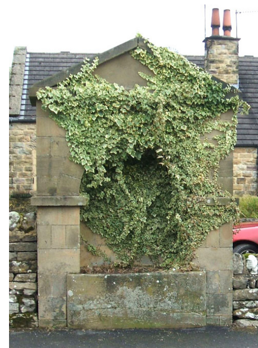
The finely jointed ashlar stonework of the village pump contrasts strongly with the dry stone walls to either side of it.
