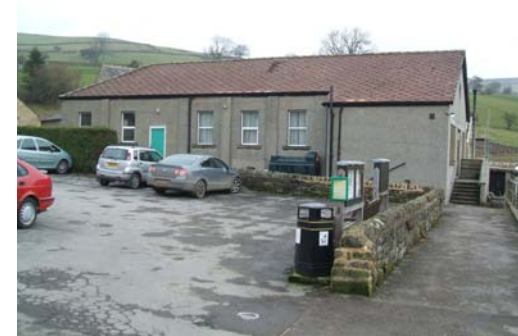
Car park adjacent Lofthouse Memorial Institute.
