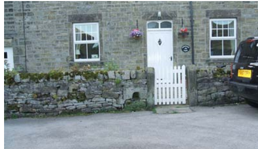
The dry stone boundary at Fountains Farm incorporates a boot scraper
