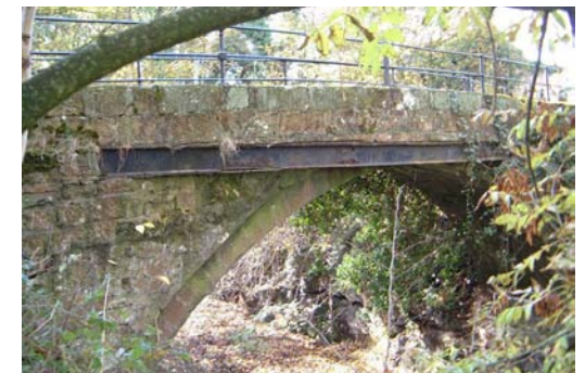
Lofthouse Bridge. Note the steel beam supporting the parapet.
