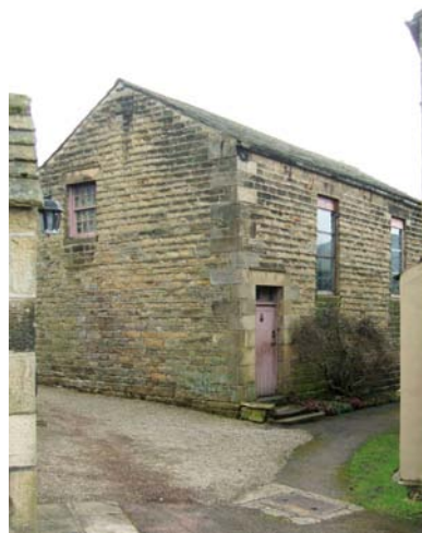
Well maintained, but seemingly vacant, the former Sunday school could be re-used.
