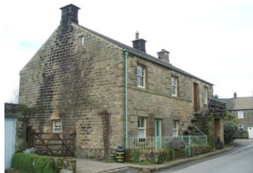
Dale Cottage is an unusually grand cottage-workshop
