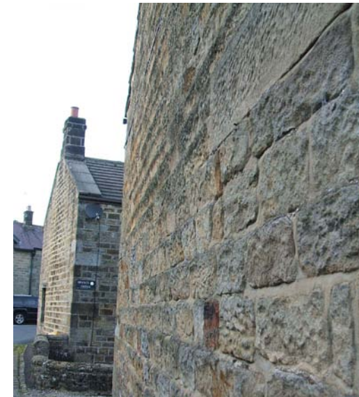
Watershot masonry is a Pennine detail
