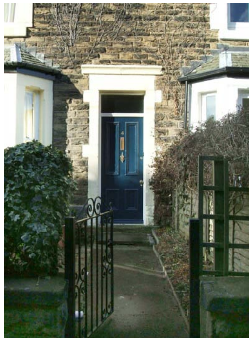
Door details at 4 Mill Lane
