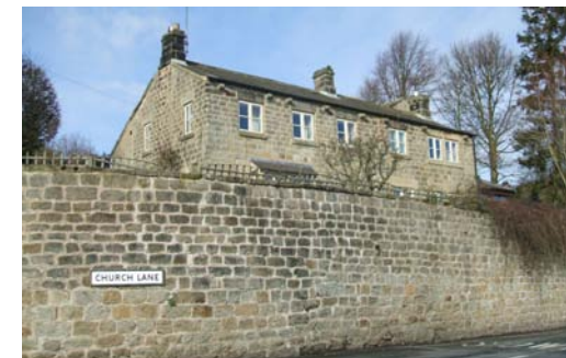
High retaining wall at Woodcock Hill
