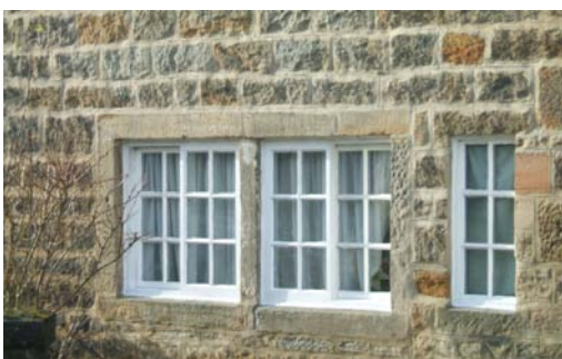
Window detail at 25 Main Street (unusually two Yorkshire sliding sash windows linked together).
