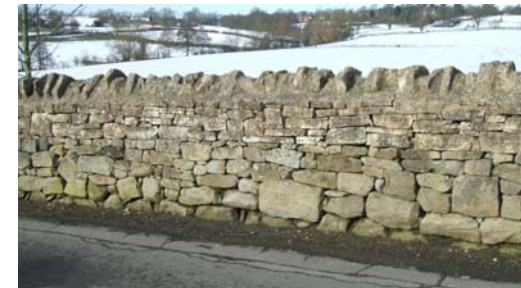
Wall opposite The Old School Room
