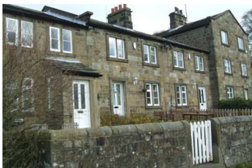
Church Row: slightly projecting stone surrounds to windows. The quoins to the corner of the gabled house and the quoins and kneeler to no.2 are visible.
