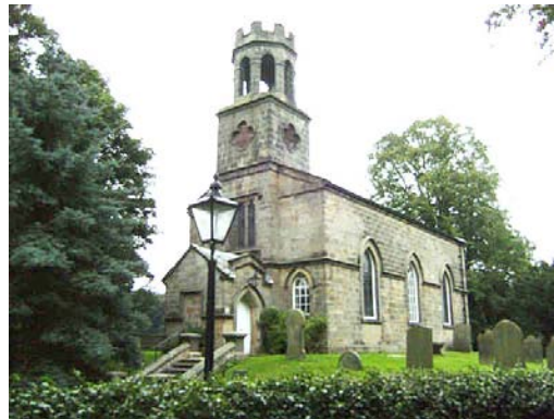
St Helen's Church: 'Gothick' decoration to a Classical building.
