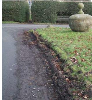
Damage to verges such as this is unfortunately widespread in the Conservation Area
