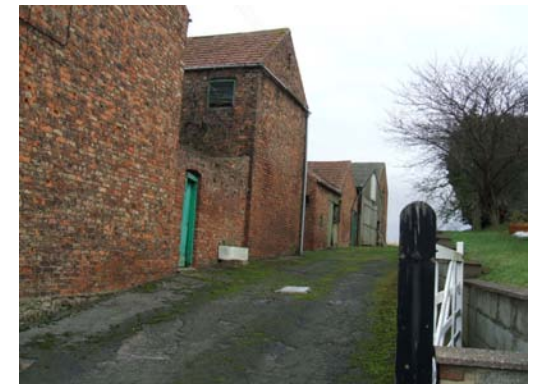
Traditional farm buildings to rear of farmhouse fronting Main Street.
