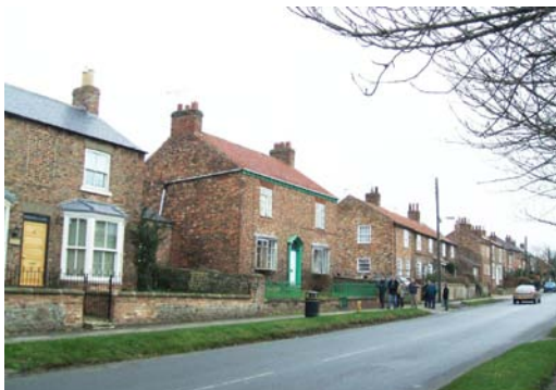
The variation in roofline along Main Street.
