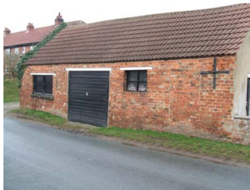
Traditional brick outbuilding associated with Pear Tree House.
