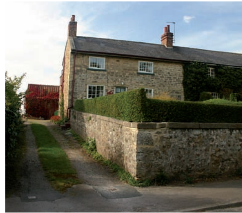
Yorkshire (horizontal) sliding sashes on Jasmine Cottage, Main Street
