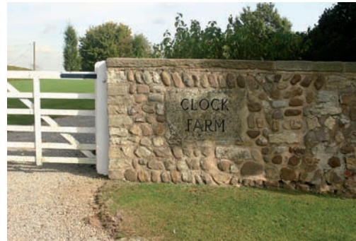
Clock Farm wall by the Main Street entrance - cobble construction with flat coping stones.
