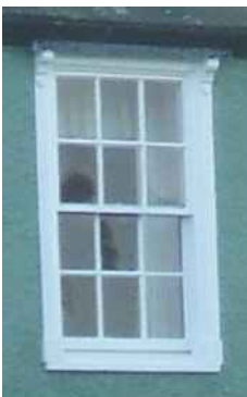
3) Tall multi-pane sash windows on a high status eighteenth century house.
