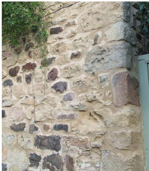
Irregular quoins and coursed rubble walling at The Old Cottage.
