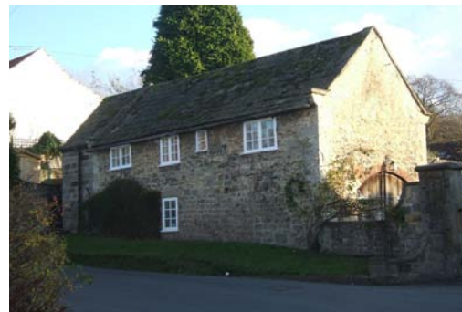
The Granary. The arched cart entrance is visible on the gable.
