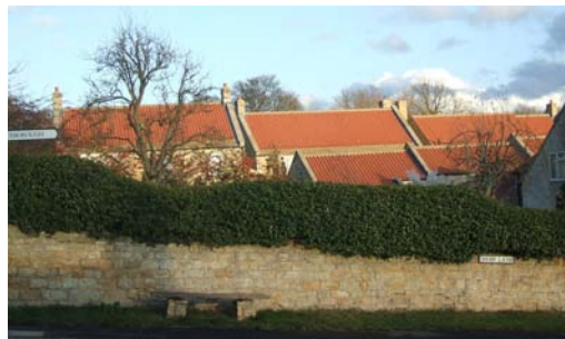
The tightly packed roofs of Manor Court.
