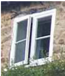
1) Timber side hung casements on a humble eighteenth century building.
