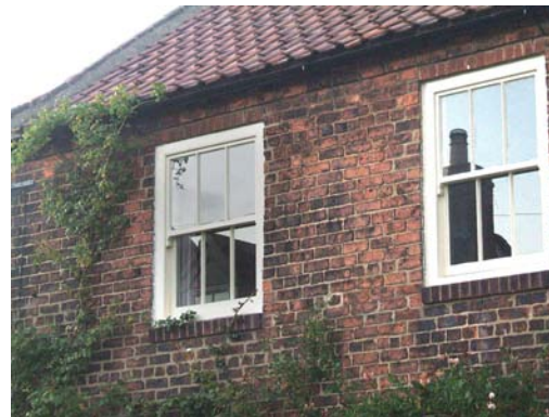
6 pane sliding sashes at Pear Tree House.
