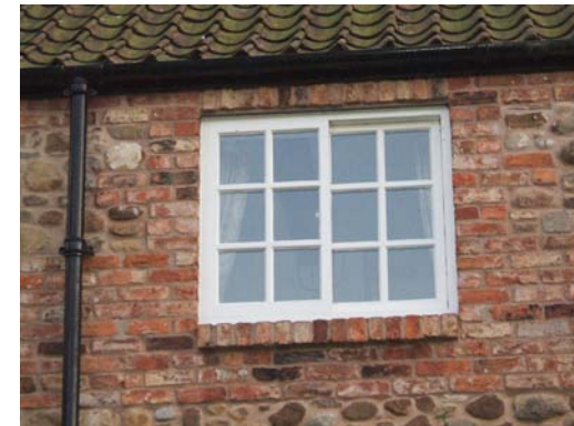
One of the few Yorkshire (horizontal) sliding sash windows in the village, at Elm Tree Cottage.
