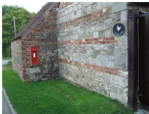
Typical traditional construction at Cottage Farm.
