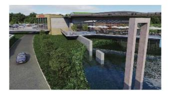
A concrete screen wall also runs from north west to south east linking both buildings and creating a defined cut through the existing landscape. The screen wall is perforated in various locations to allow access through and into the hotel, delivery yard and amenity building before stepping down through the external seating terrace and terminating in the ornamental lake to the south of the amenity building.
