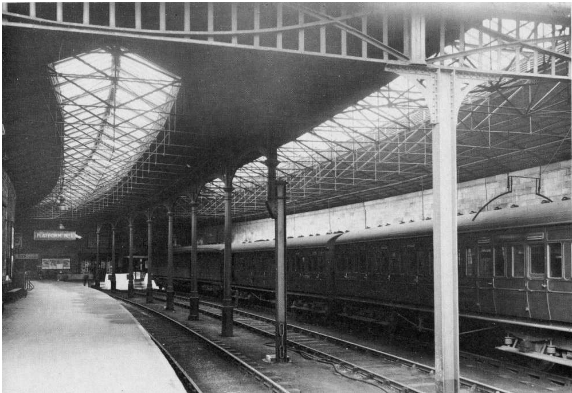
Interior of Trainshed
