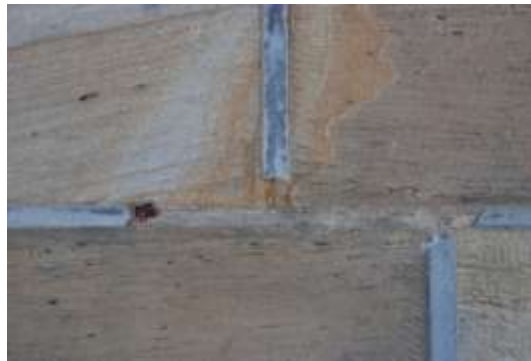
Strap pointing within Portico
