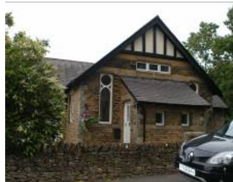
Local interest buildings Right Former Methodist Chapel, Ruston
