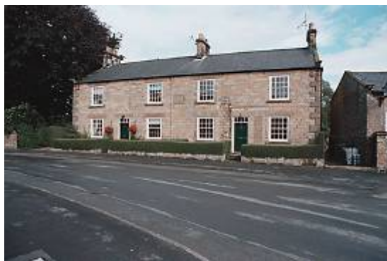
Listed buildings – 23-24 Wykeham
