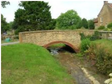
Left Ruston Bridge © J Thomas
