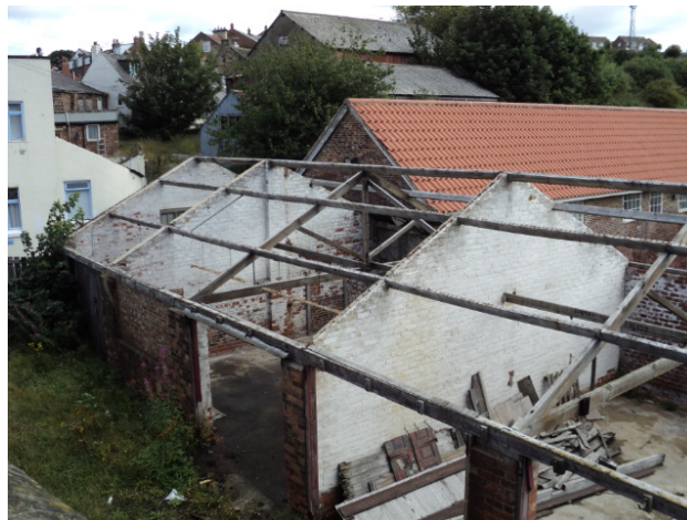
Derelict buildings on Raft Yard
