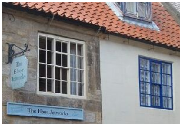
Above and below - the design of window known as The Whitby Composite sash
