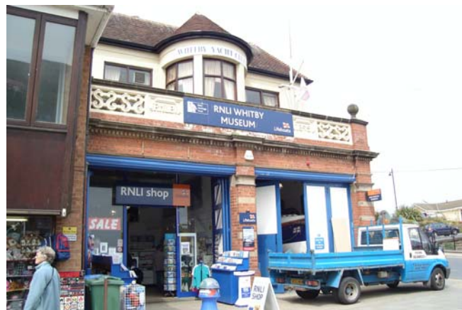
Former lifeboat house
