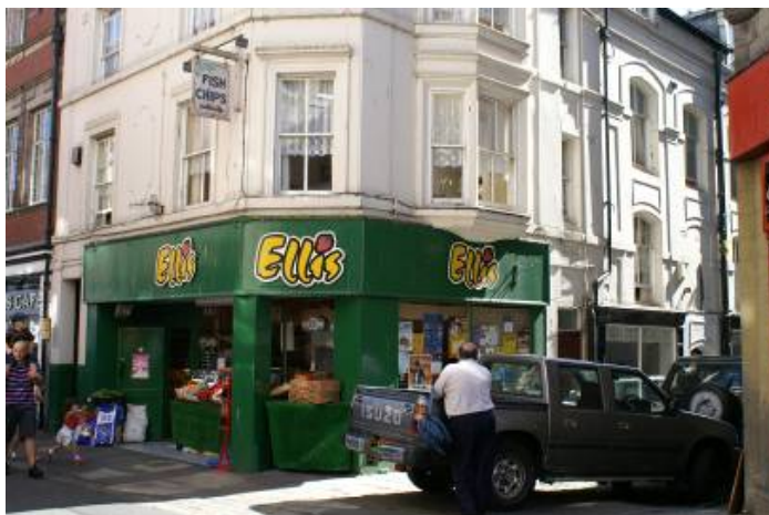
Example of a poor shop front which fails to respect the robust architectural qualities of the building above
