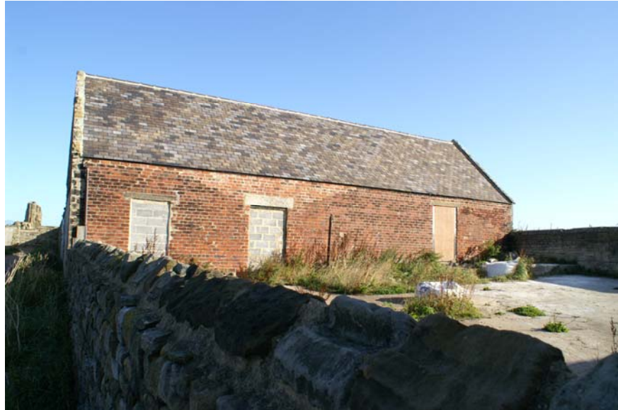
Disused buildings at Abbey Lands Farm
