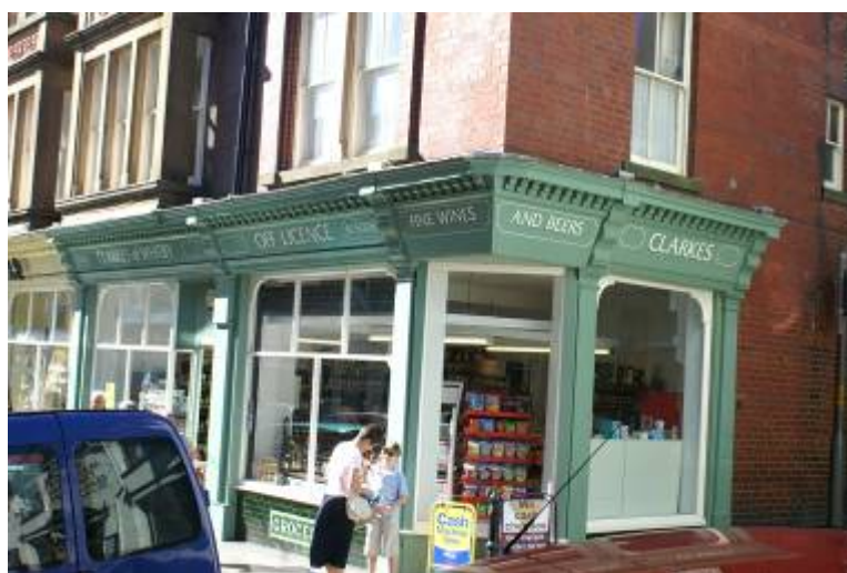
Example of one of several shop fronts in Skinner Street falling in the Excellent category as it retains a considerable amount of original detail such as glazed brick stallriser, decorative fascia and entablature and console brackets
