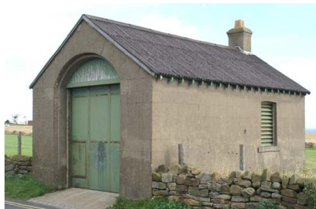
Former rocket post house
