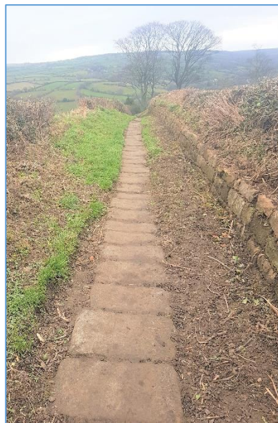
Two photos showing examples of the work carried out by the Probation Service Community Payback Scheme on Featherbed Lane
