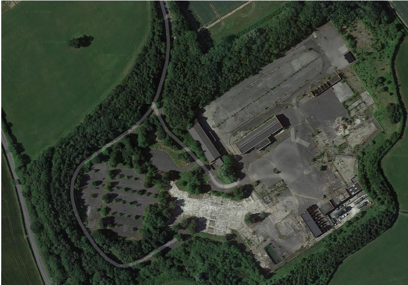
Appendix C – Aerial Photo (source: Google Maps – aerial photo 15 th July 2020)
