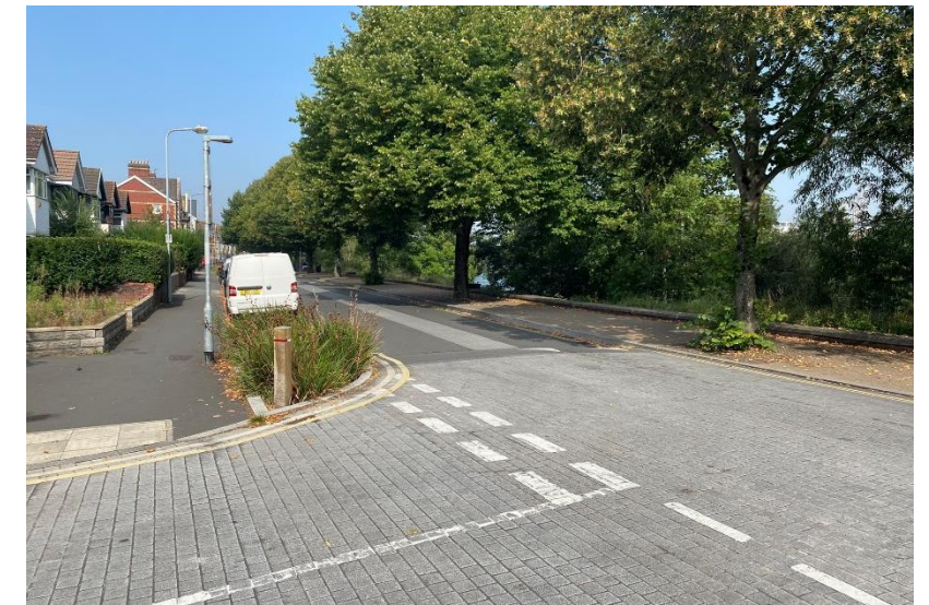
Figure 4.6. Buildouts with SUDs
