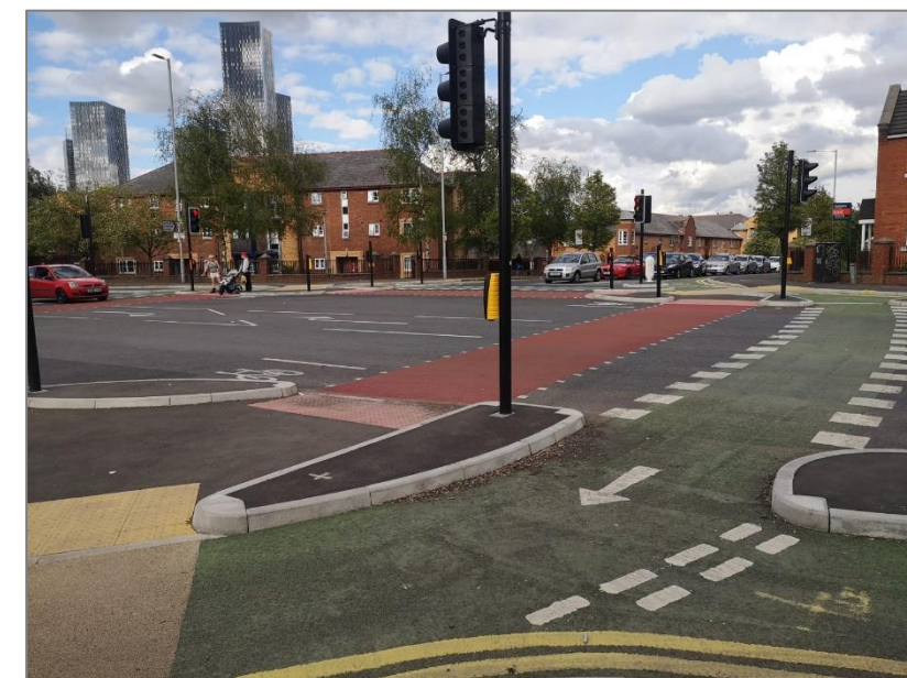
Figure 3.14. CYCLOPS signalised junction
