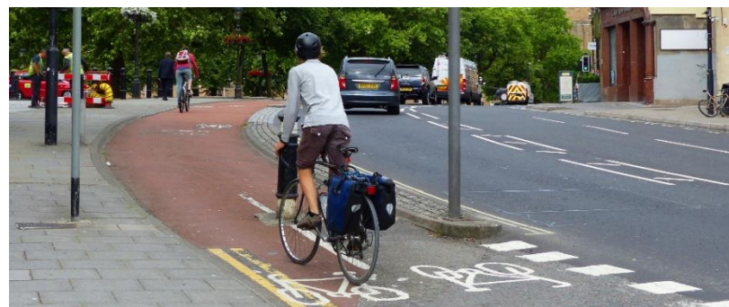
Figure 3.7. Segregated cycleway (carriageway height)
