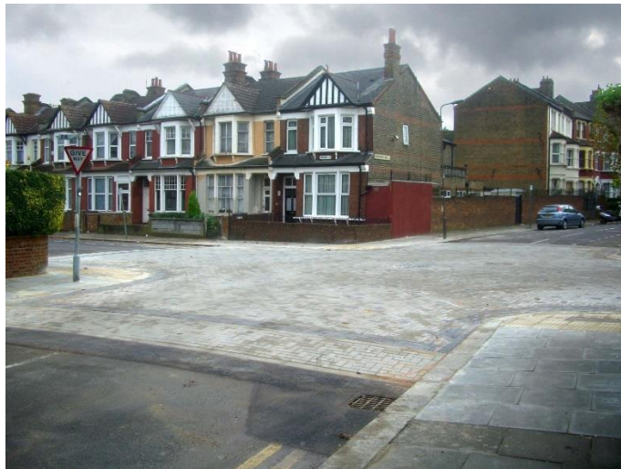
Figure 4.7. Raised table junction
