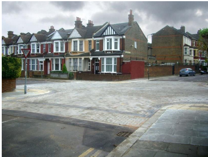
Figure 4.8. Raised table junction
