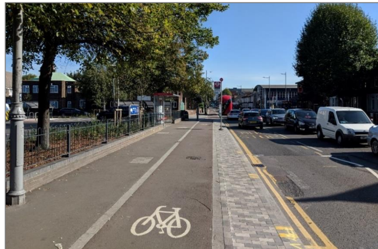
Figure 3.10. Stepped cycle track (intermediate height)
