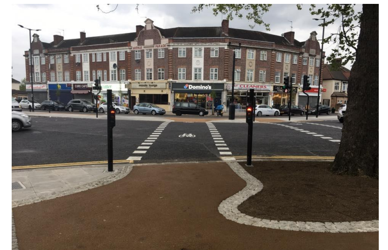
Figure 4.7. Improved signalised junction (Enfield)
