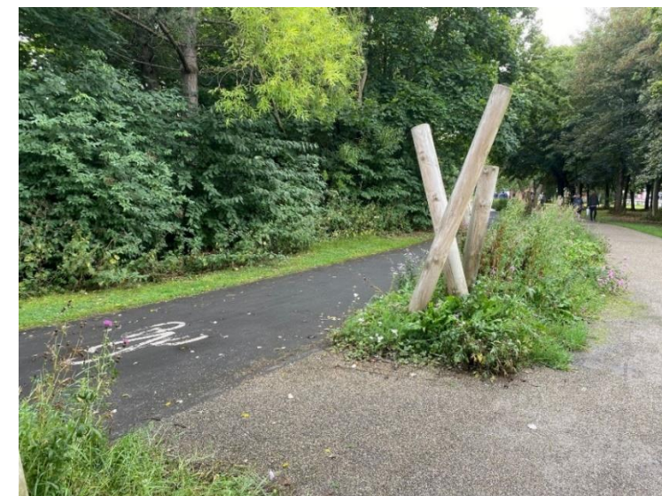
Figure 3.9. Greenway (segregated cycle / pedestrian facilities)
