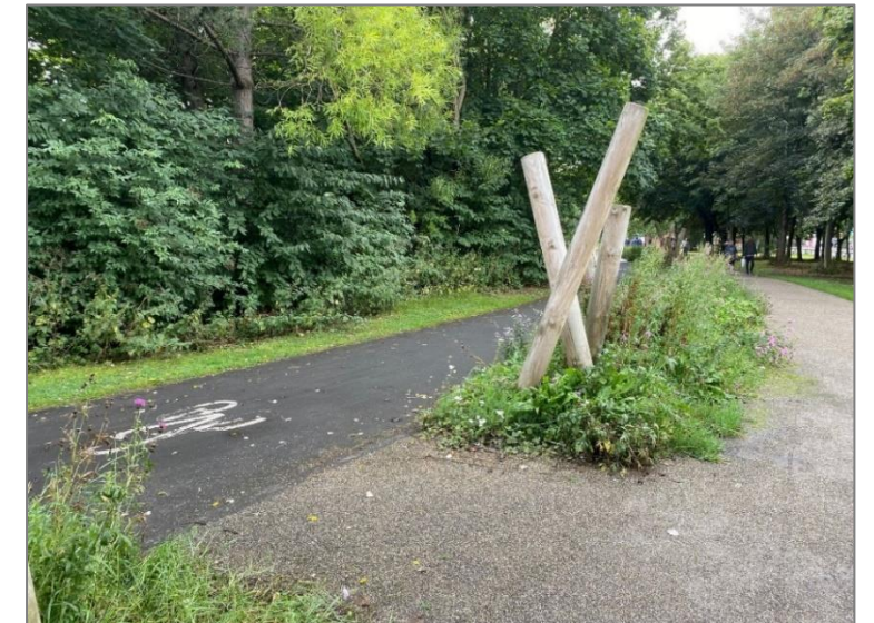
Figure 3.11. Greenway (segregated cycle / pedestrian facilities)
