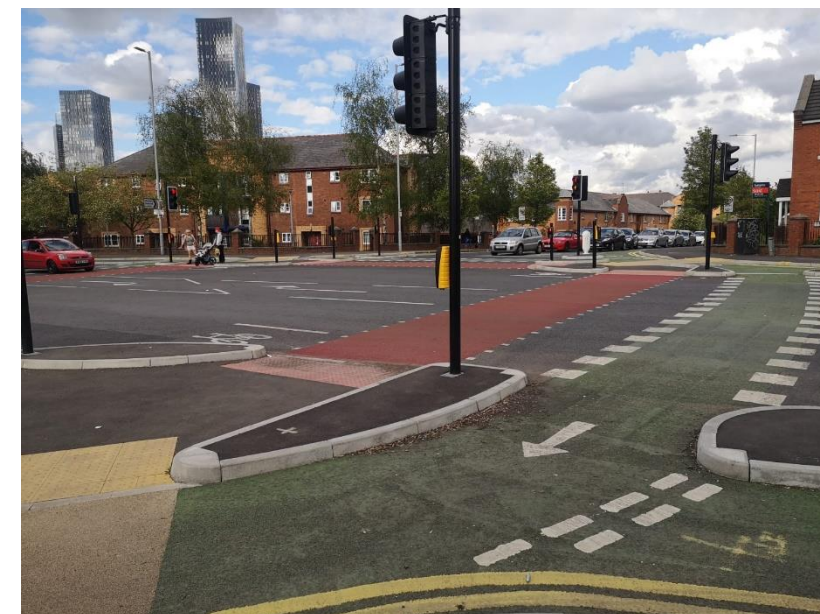
Figure 3.12. CYCLOPS signalised junction
